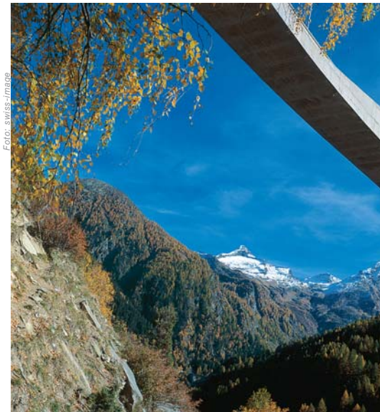
A ponte Ganter no Simplon Ganter bridge on Simplon Pass
